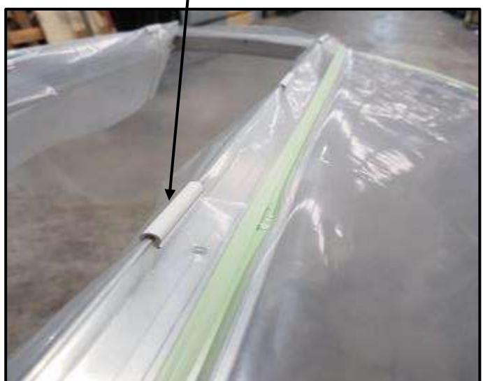
(Pic V5) shows omega clip fitted to upstand – which holds the tail of the cover behind the vent rail and acts as a flashing
