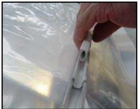
Tap the bead into place
