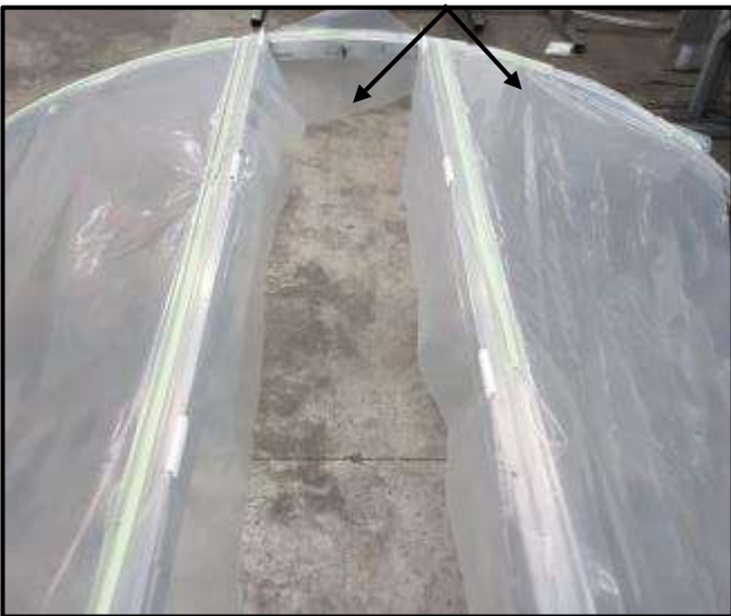
(Pic V4) Shows cover cut away and 100mm piece of Lockstrip insert + clip to hold the end in place
