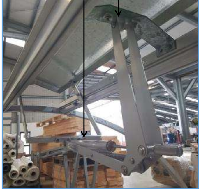
Locate pivot foot to handle and bracket as shown
