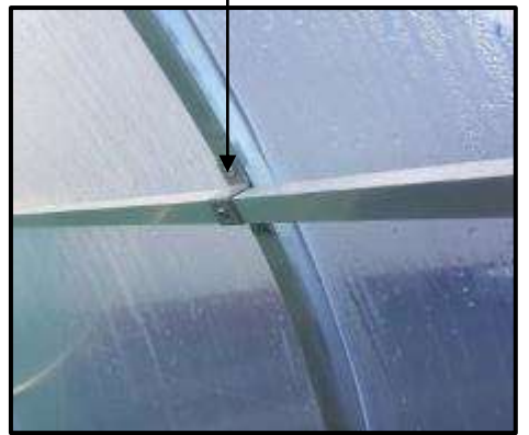
Saddle holding side purlin in place (P3)
