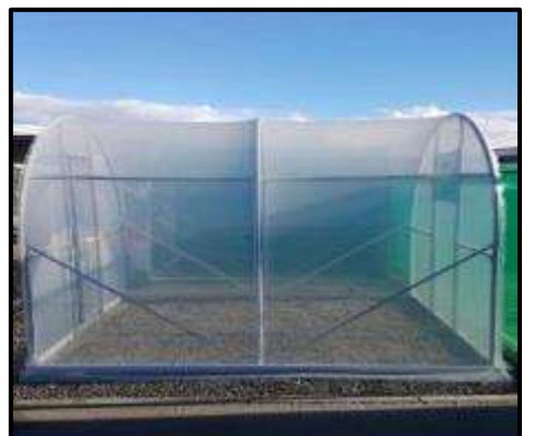
Side view of purlins fitted
