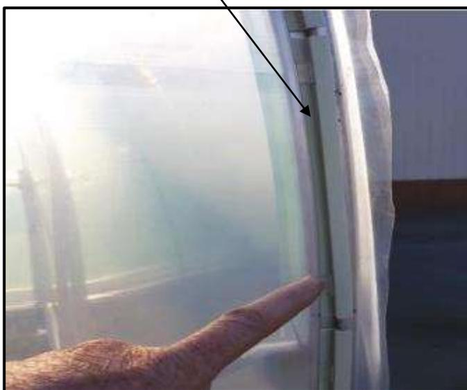
(Pic L2): Shows the positioning of the covering (red), Insert (green) and Lockstrip clip (Black)
