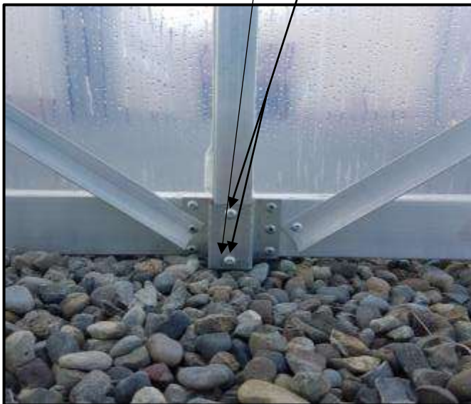
(Pic SBS1) - Side base rail saddle (Secure these internal hoop screws after the cover installed)
