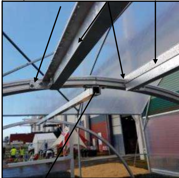
(Pic V1) Vent "L" Bracket x 4, Vent rails Vent Upstands
