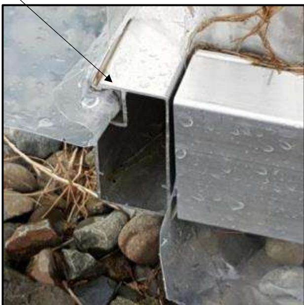
Corner side base rail finishes flush with end rails (Pic BR1)
