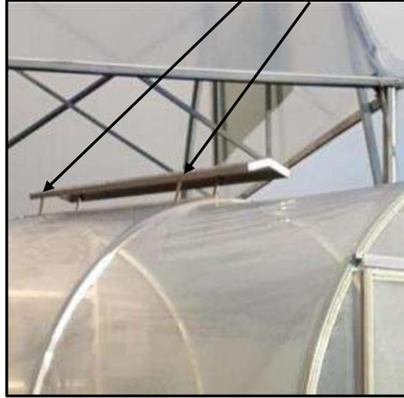
**Note:** The ridge beam purlin should be removed from the vent location space; the vent rails replace the ridge purlin in the vent space.
