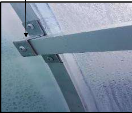
Purlin ends (P1)
