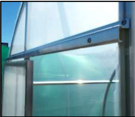
Exterior view of door track (Pic D1)
