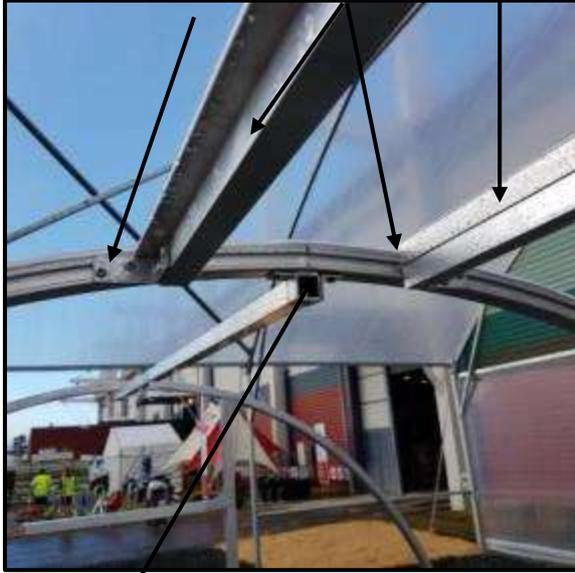
(Pic V2) Roof vent cap and Vent arms + Handle
